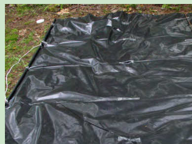
Construction of a 6-mil polyethylene benthic barrier.
