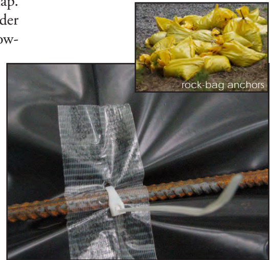
Benthic barriers must be weighted to hold the tarp like material in place. Common methods are rebar attached with electrical ties, rock-bag anchors, and bricks.
